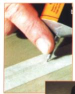
With one hand press the needle of the tube firmly inside of the seam and pull along. With the other hand dose Cold-Welding Liquid so that an approx. 5 mm wide line appears on the masking tape.
